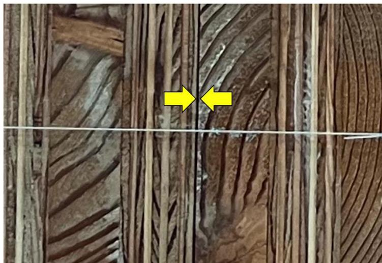
**Fig. 7.** The space created between the lamination of nail-laminated timber by concrete pouring
