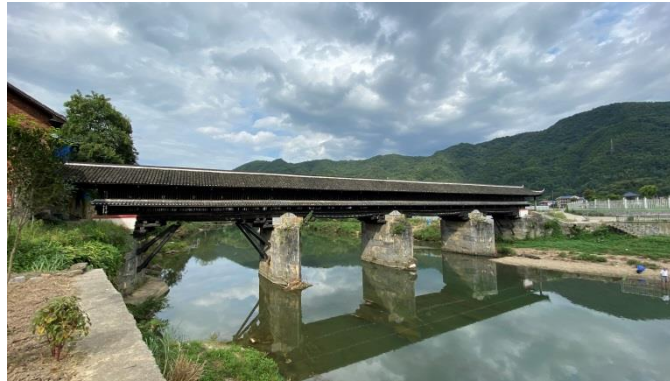
Fig. 6. Photograph of Shiyi Bridge
