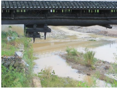
(a) Cantilever system on abutment
