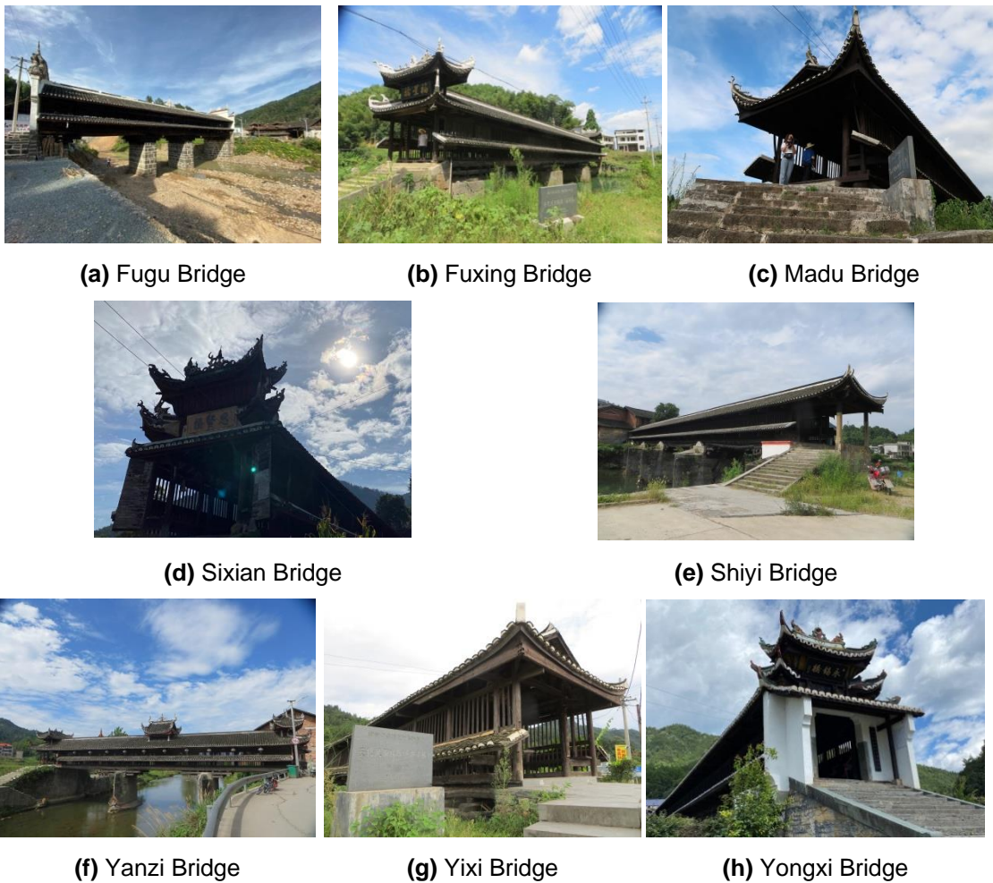
Fig. 16. Roofs of Anhua covered bridges
