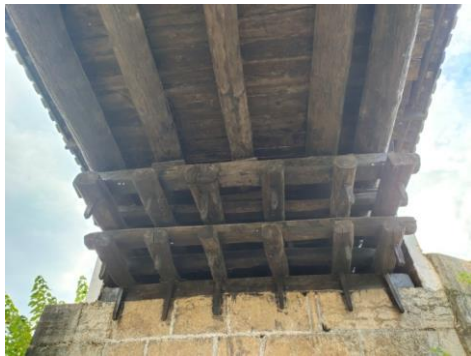
(c) Detail of cantilever system
