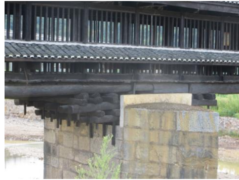
(b) Cantilever system on pier
