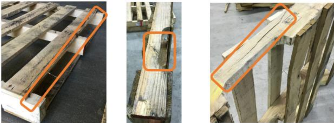
Fig. 2. Representative picture of missing wood (left), break (middle), & split (right) damage modes
