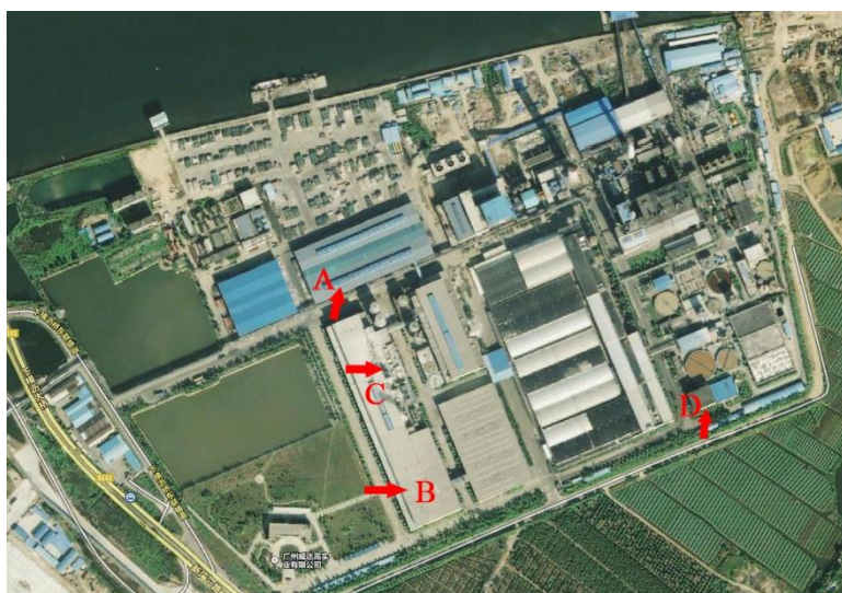
Fig. 2. Overview of the plant and the sampling locations: (A) waste paper sorting room, (B) papermaking workshop, (C) vacuum pump outlet, (D) office area
