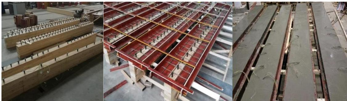
Fig. 1. Construction of the TCC
